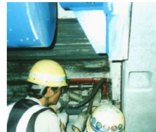
pulling pipe out
