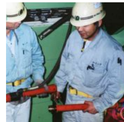
Pulling Mixing-nozzle out
