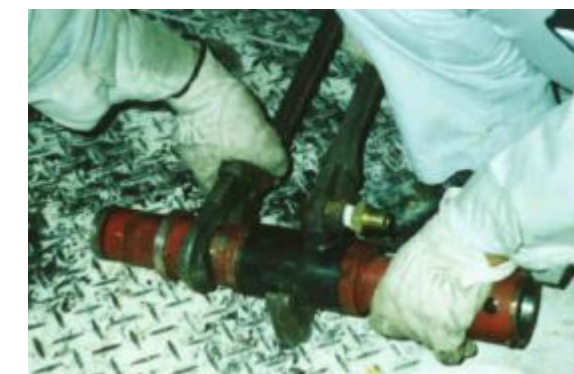
Maintenance of Mixing-nozzl
